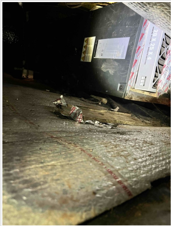
Media door on ground
